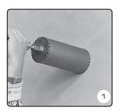
Use a core drill with min. dimension Ø102mm for Fresh 100 and Ø150mm for Fresh 100dB. Drill from inside to outside. Drill the hole so that the pipe slopes slightly downwards.
