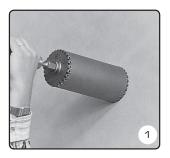
Use a core drill with min. dimension Ø86mm for Fresh 80 and Ø 150mm for Fresh 80dB. Drill from inside to outside. Drill the hole so that the pipe slopes slightly downwards.
